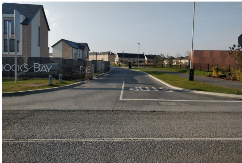
Figure 13.4: New Primary Access looking from Station Road.
