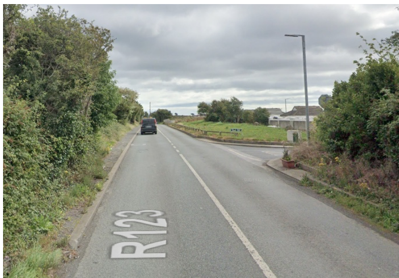
Figure 13.5 Moyne Road R123 looking East (Source Google Maps).
